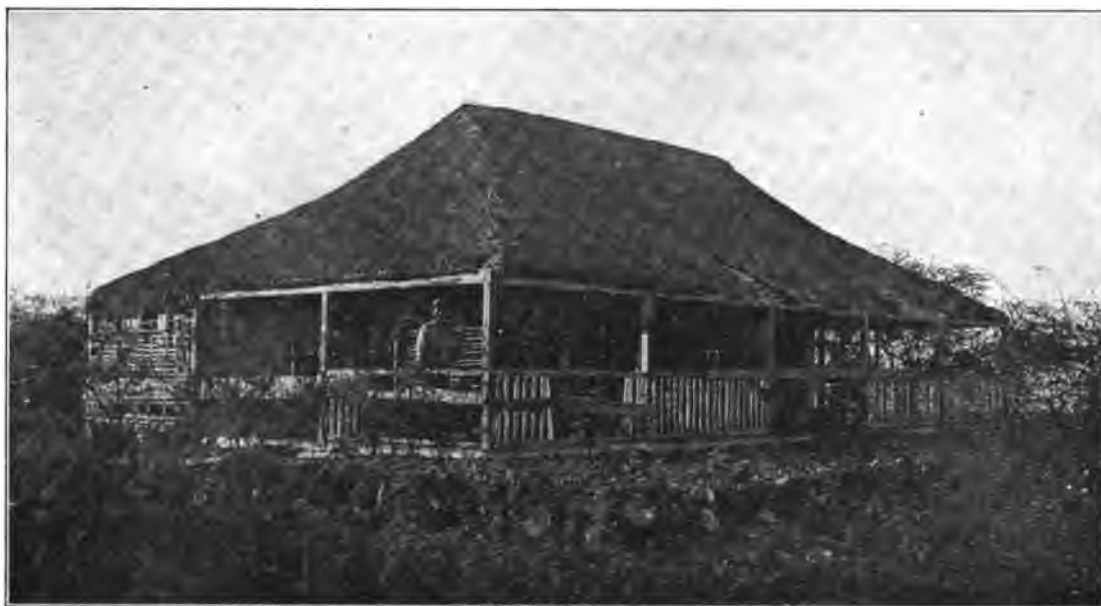
FIG. 95. HOUSE OF KAMEHAMEHA V AT KAUNAKAKAI.
